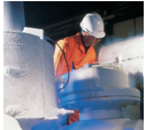
Pipe freezing allows maintenance to be carried out on-line
