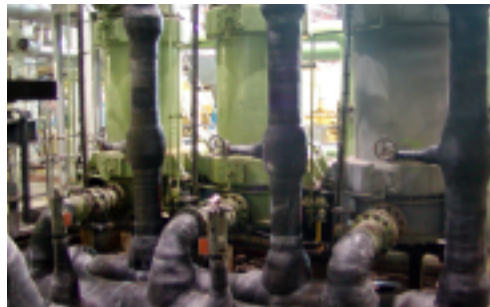
Repairs to seawater cooling system
