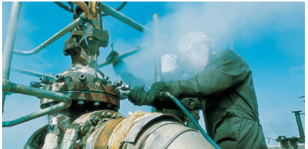
Peened wire repair
