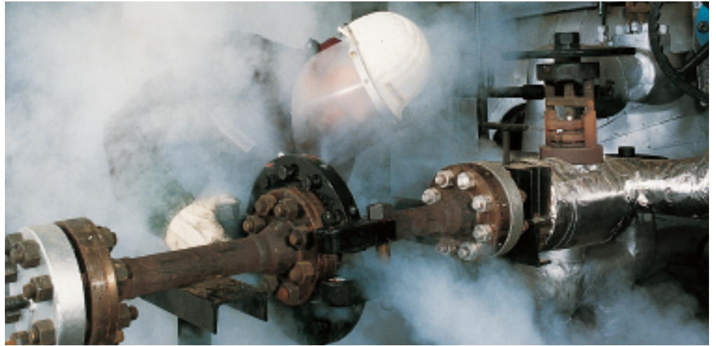
Fitting a ring clamp
