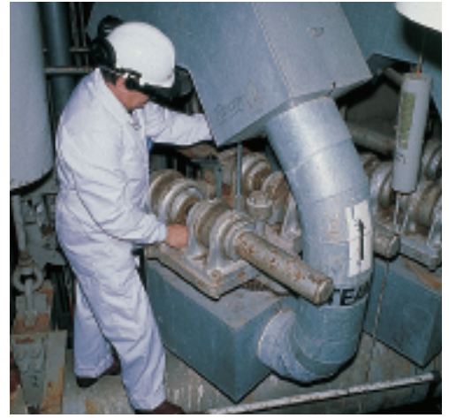
Testing a Torsion Bar Relief Valve
